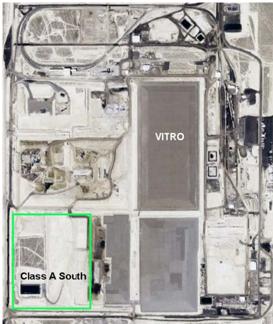
Figure 2. Disposal and Treatment Facilities operated by EnergySolutions.
